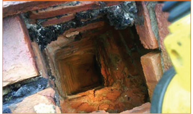
Image 1: Chimney in poor condition
