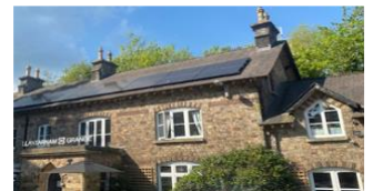
SOLAR PANELS AT LLANTARNAM GRANGE- ARTS CENTRE, CWMBRAN
