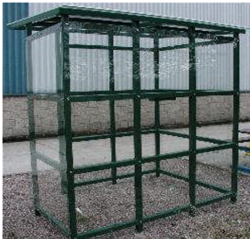
Non Compliant bus shelter
