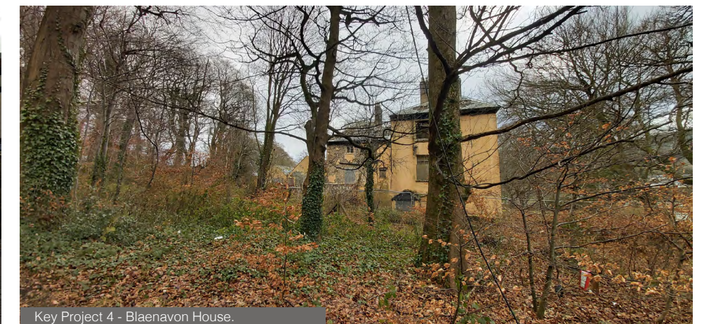
Key Project 4 - Blaenavon House.
