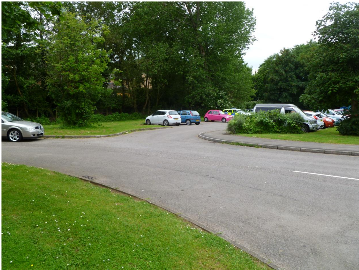
Image 14: Car park adjoining the Dowlais Brook, Two Locks Road after the event.
