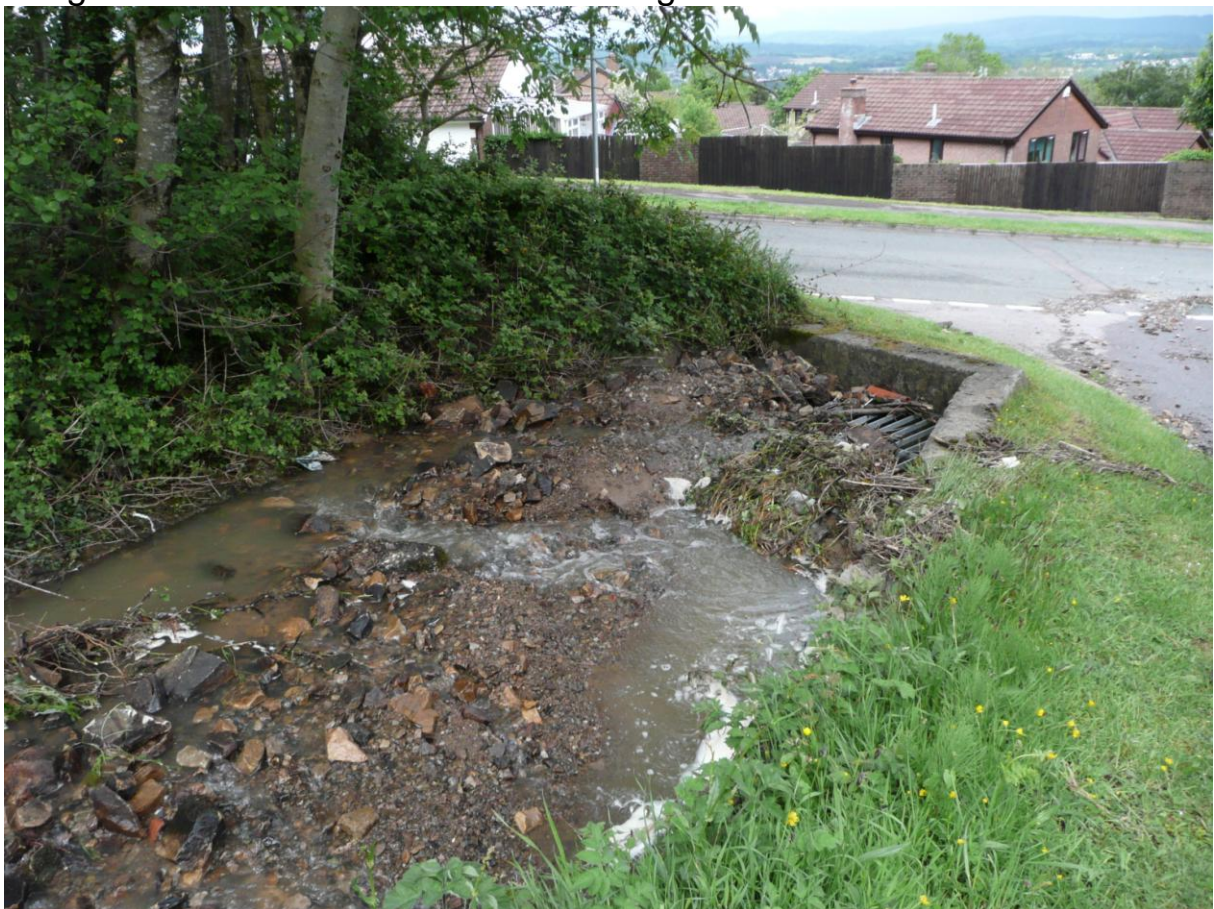
Image 5: Culvert No 134 after the flooding event
