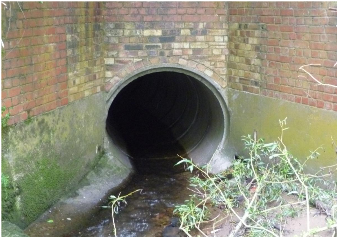
Image 1: A 1.5m Diameter culvert designed for the 1 in 100 event return period approved by the National Rivers Authority in 1992/3.
