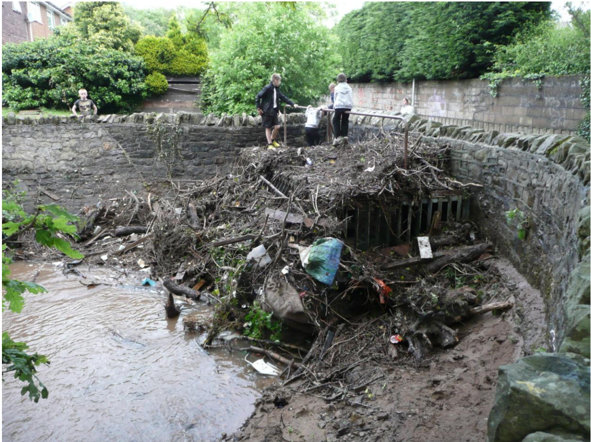
Image 4: Culvert No 95 after the flooding event
