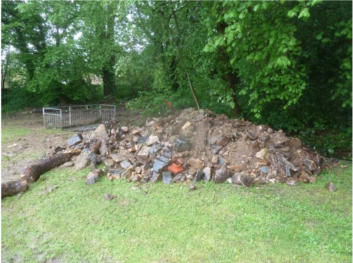
Image 8: Material removed from Culvert 94 totalled 35tonnes.
