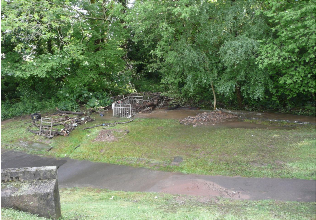
Image 6: Culvert no 94 after the flooding
