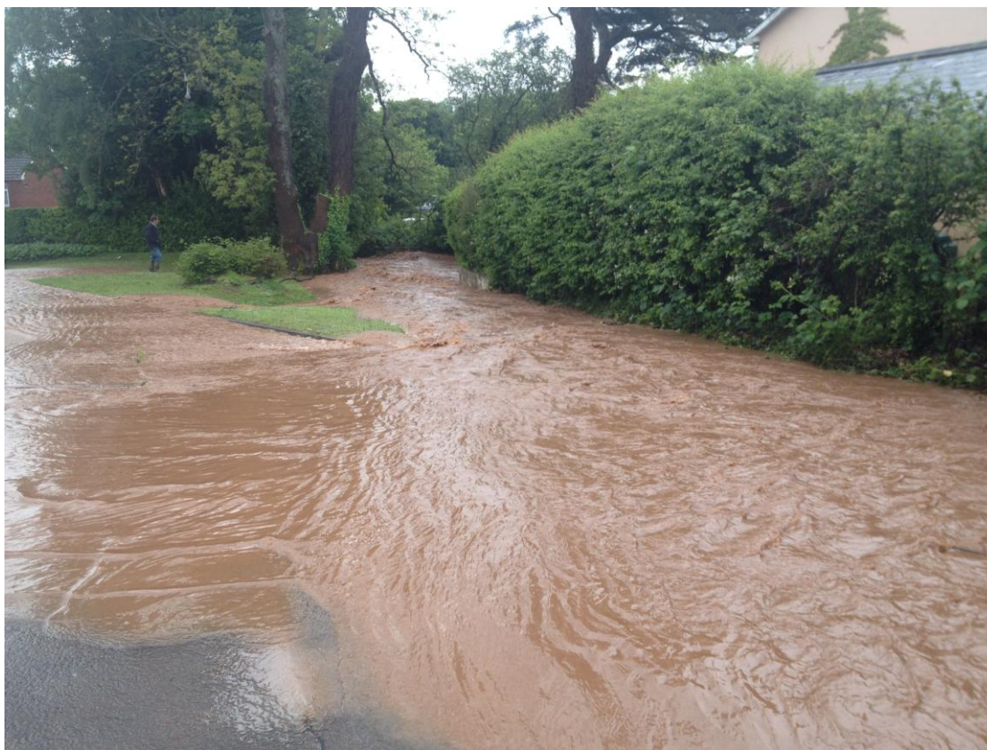
Image 15: Hollybush Close flood route after the rainfall event surcharging from Culvert 112
