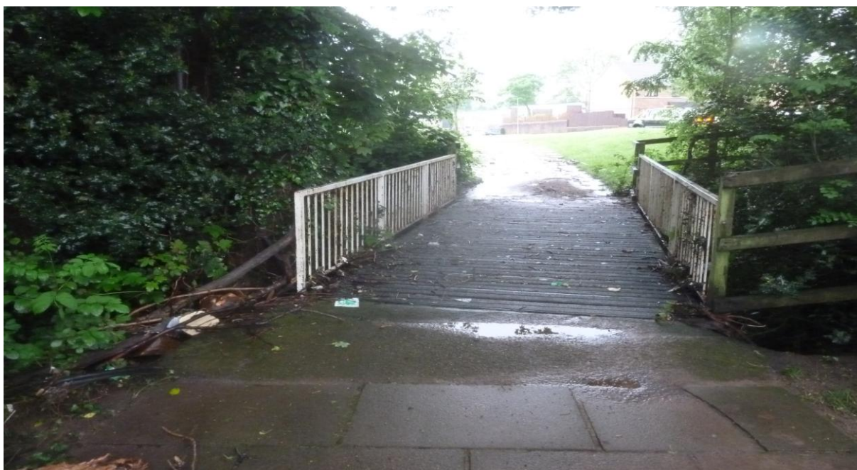
Image 16: Open footbridge that allowed the flow of water to travel across.
