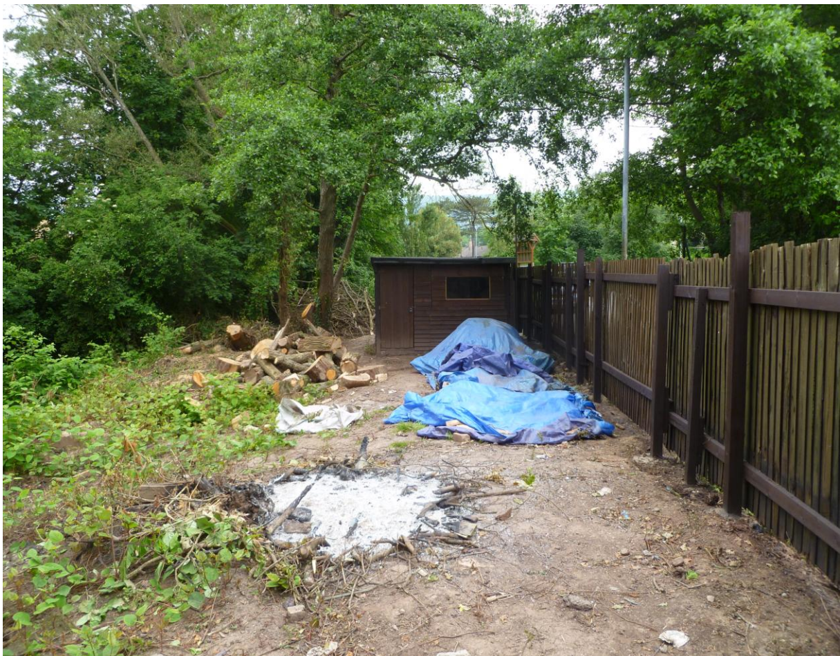
Image 11: Banks of Dowlais Brook above the inlet near Gifford Close (Privately owned and overseen by NRW).
